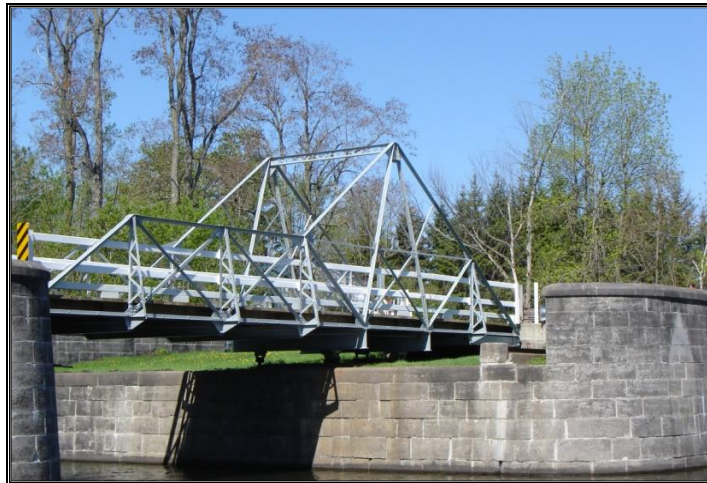
The Swing Bridge at Burritt's Rapids
