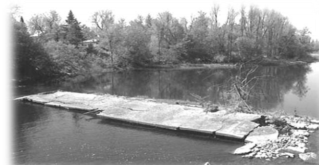
*Burritt's Rapids Dam
