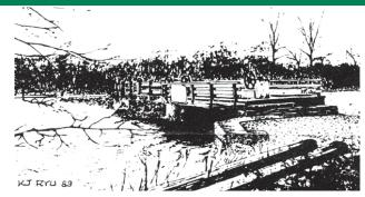
Like Colonel By in the early 1800's, Parks Canada uses these dams to raise or lower water levels. This is done by using winches to adjust the number of stop logs in the dams. These water levels are regulated to meet a wide variety of needs, from navigation and natural habitat conservation, to hydro-electric and municipal water supplies. In spring when there is more water flowing, more logs are removed.
